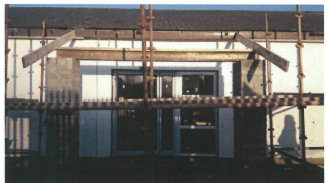
Porch going up over new entrance to hall.
