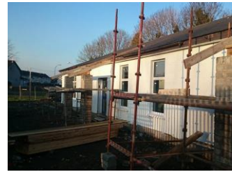
New porches over old entrance and new hall entrance going up.
