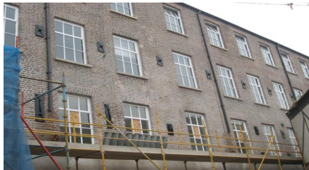
Window replacement is underway at Conway Mill.
