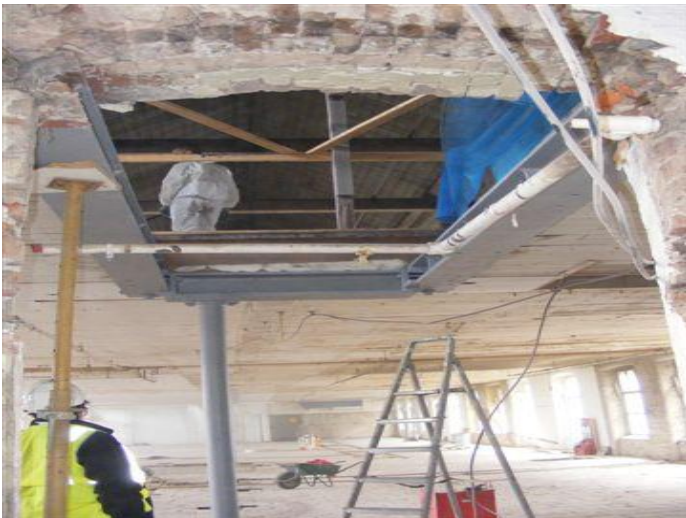
Third floor renovations – Old Mill, May 2009
