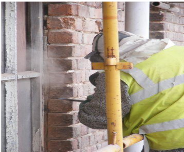
Repointing on the third floor
