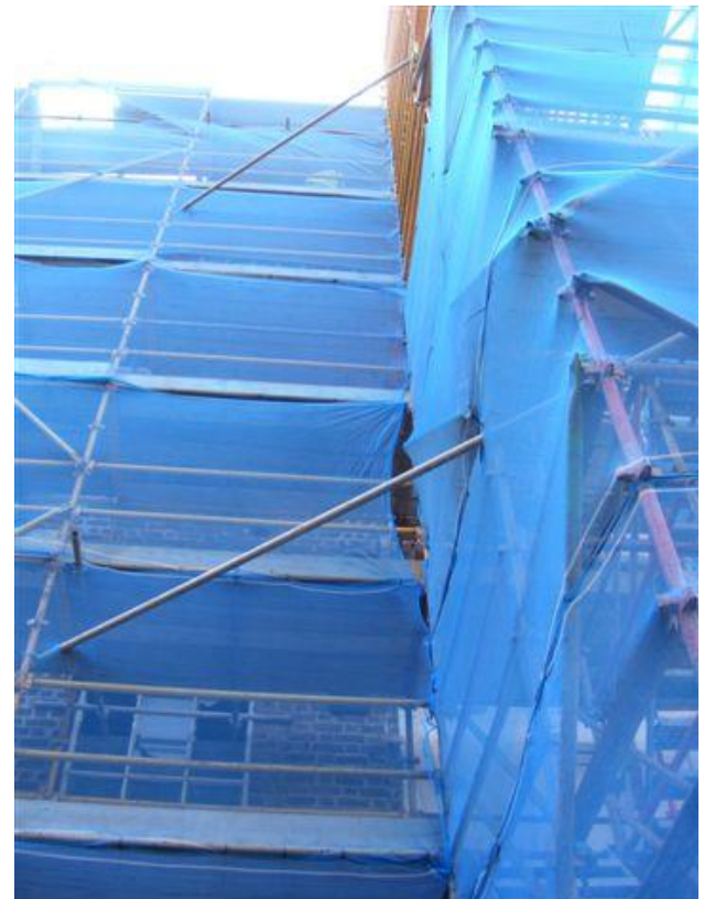
Scaffolding on the Old Mill – May 2009
